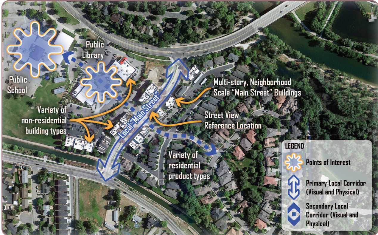
Source: Google Earth Pro, Bown Crossing Mixed Use Area, Boise, Idaho 43°34'27.13"N, 116° 9'17.73"W. [Accessed June 2023].
